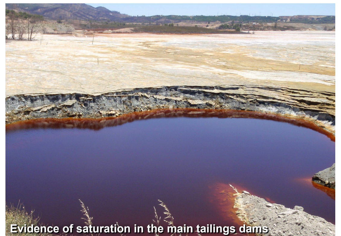
Evidence of saturation in the main tailings dams
